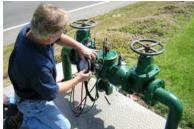
BFP Testing is an annual requirement by GWA per Title 28 Public Utilities GAR to ensure the continual proper operation of a backflow preventer. BFP testing is currently enforced by GWA on to its customers who have BFP's Installed at the GWA Meter as also required by GWA. These BFP testing for GWA customers is only performed by 3<sup>rd</sup> party individuals/contractors per GWA.
